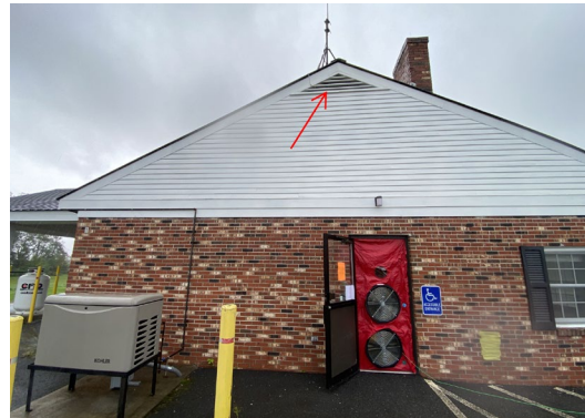
Attic venting in the gable end of the roof.
