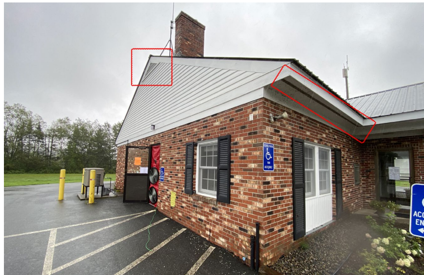
Looking at a gable vent and soffit venting on the exterior.
