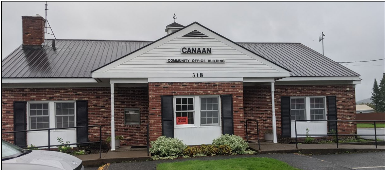
Figure 1: Building exterior (north façade)
