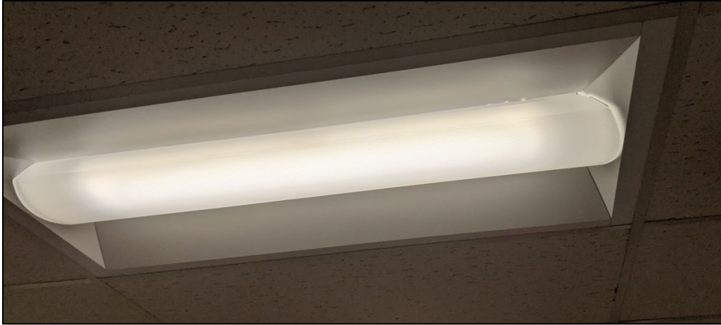
Figure 2: Recessed LED troffer
