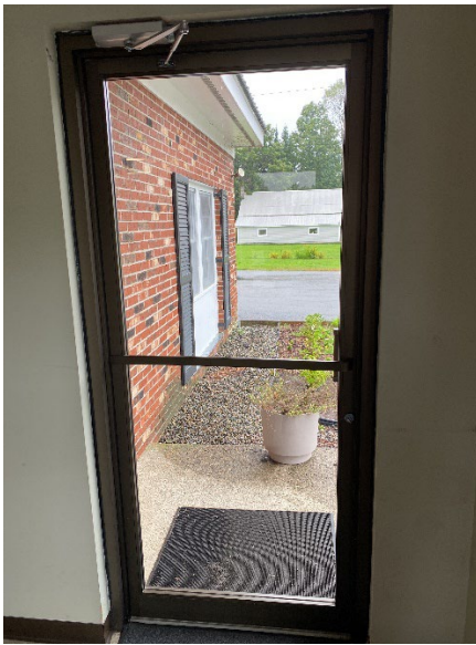
One of the main entry vestibule doors, similar to the side entrance where the blower door setup was installed.
