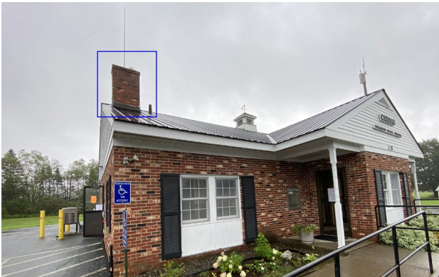
Chimney where mechanical systems exhaust.
