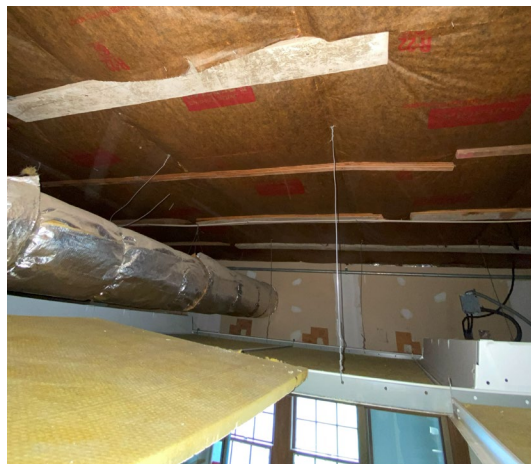
Looking above the ACT, there is a plenum space for electrical and ductwork, then the faced fiberglass insulation is visible in between roof trusses (facing is stabled to the bottom of trusses).
