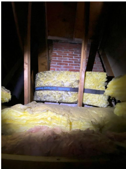
A view of the chimney inside the attic, partially wrapped with fiberglass insulation. Attic access did not allow closer inspection of this area.
