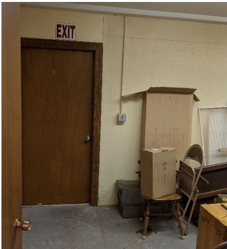
A view of the door in the basement that leads to the exterior bulkhead.
