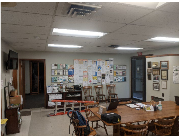
A view of the ACT grid at the first floor ceiling. This was consistent on the first floor except for the vestibule, which had a drywall ceiling.
